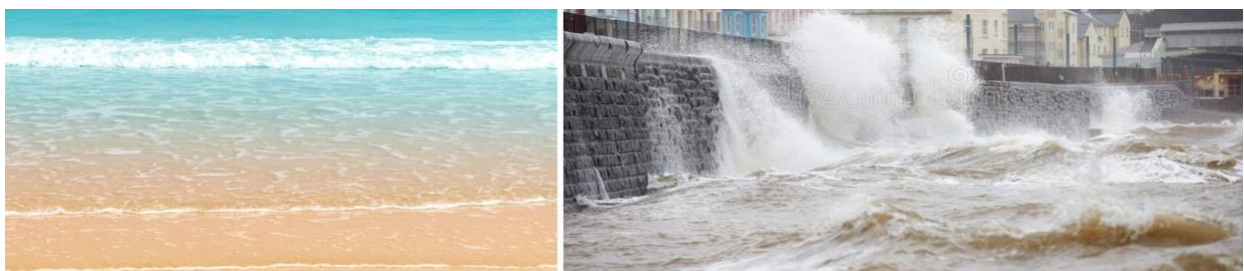
Fig 15. Waves breaking on gently sloped shore (left) opposed to hitting a sea wall (right).
